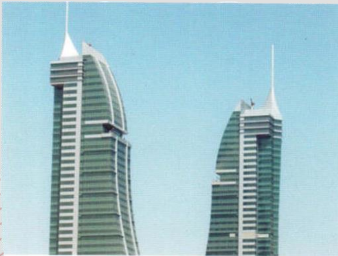
Bahrain Financial Harbour Installation of fire fighting and air conditioning systems in multiple shops
