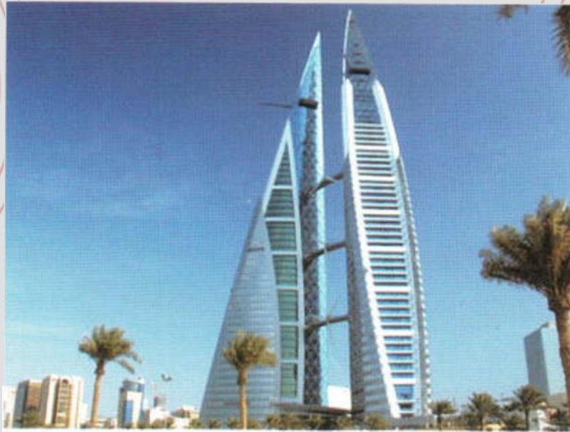
World Trade Center Fitness First Health Center Installation of air conditioning system
