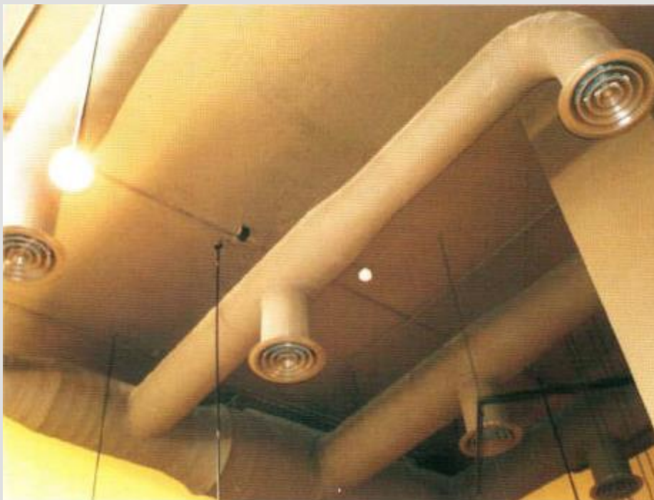
Juffair Skyview Installation of air conditioning system
