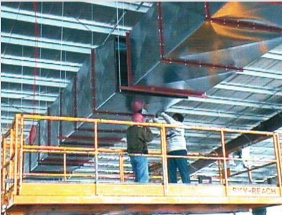
West Point Home Spinning Unit Installation of air conditioning system
