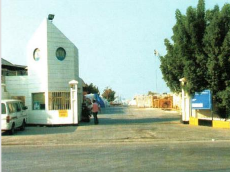
Manama Textile Mills Installation of air conditioning system
