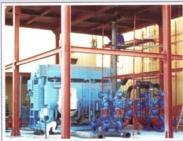
Tubular Shop Installation of air conditioning system
