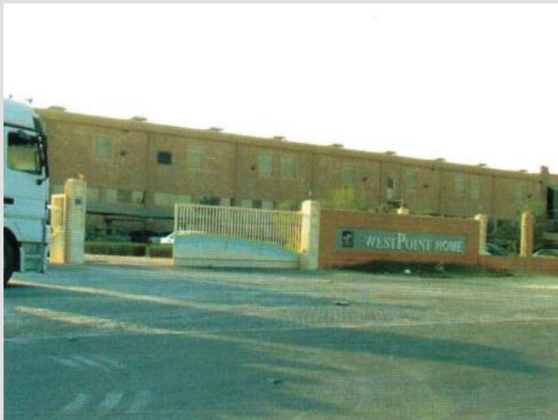
West Point Home Installation of air conditioning system
