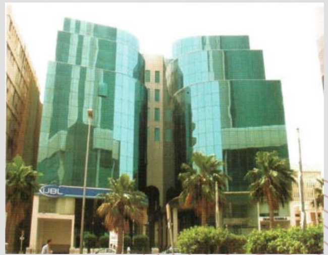
Twin Tower for Royal Court Installation of air conditioning system
