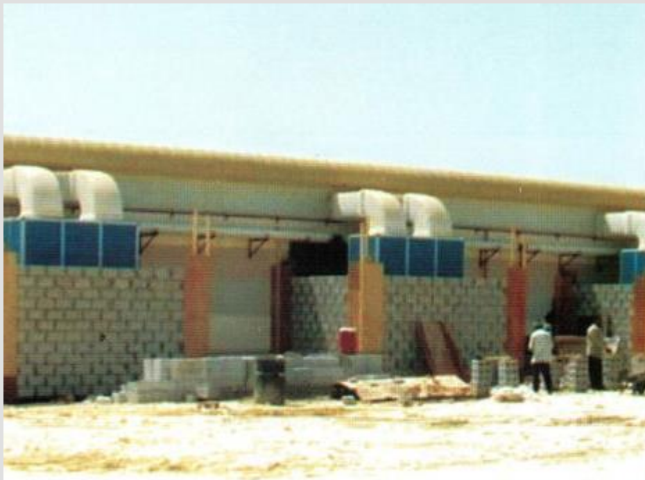
West Point Home Processing Unit Installation of air conditioning system
